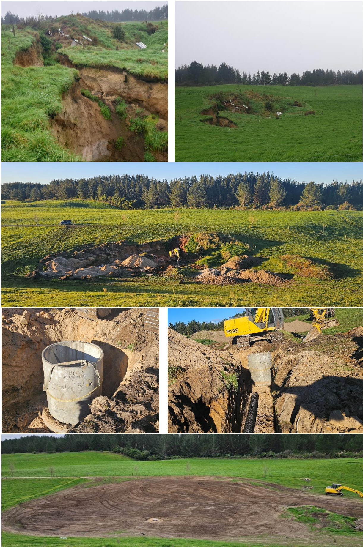
Figure 3: The before, during and after of the Tuarua tomo repair. Paddock has since been regrassed.
