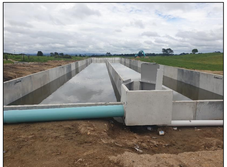
Figure 5: New effluent pond and weeping wall for solids separation on Tuarua.
