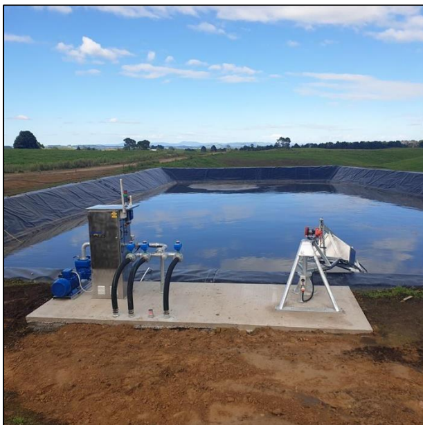
Figure 5: New effluent pond and weeping wall for solids separation on Tuarua.
